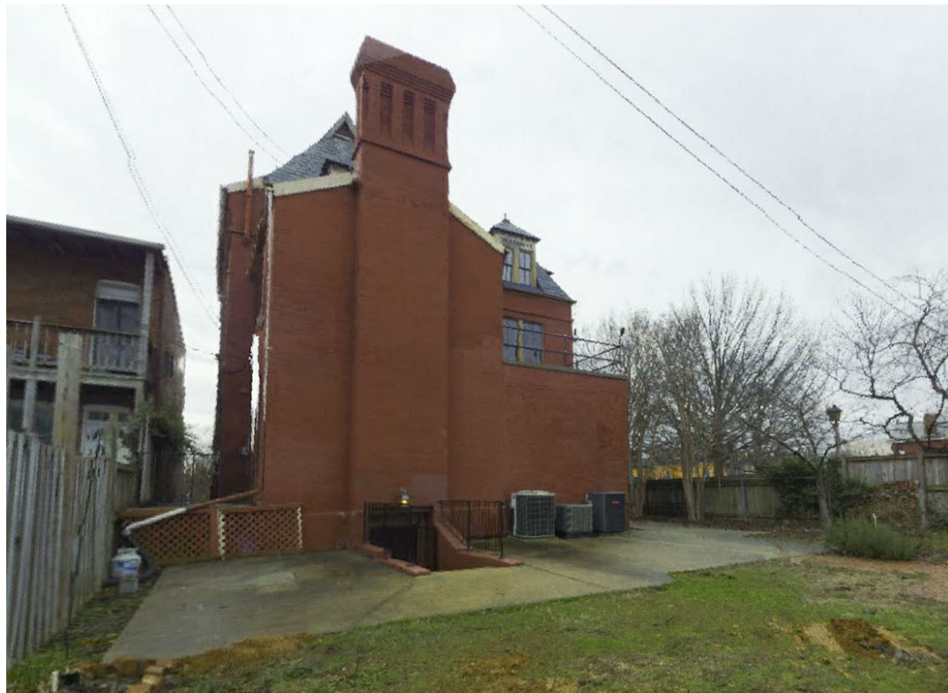
REAR YARD LOOKING SOUTHWEST
