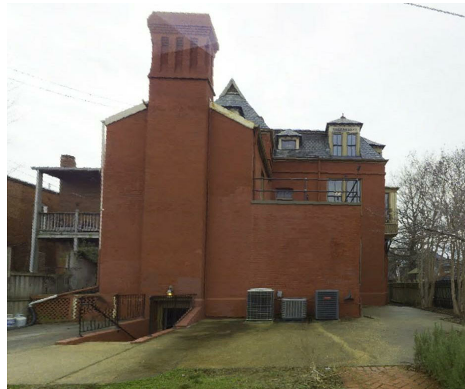
REAR YARD LOOKING SOUTH
